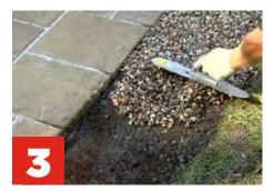
Trowel the mixed riverstone on the surface desired, with a minimal thickness of 13 mm within 20 minutes after mixing
