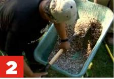
GATOR ROCK BOND KIT Mix one 473 ml container of GATOR ROCK BOND with 100% dry clean riverstone (18.2 kg) provided for 4 minutes.
