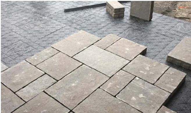
"Much easier and faster to lay the paver down."
