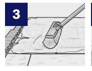
**3** Sweep off excess EUROSTONE BOND from the paved surface, first with a hard-bristle broom, then a soft-bristle broom. Take care to leave the height of EUROSTONE BOND at least 3 mm below top of natural stone pavers surfaces.
