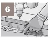
Install Gator Tile Edge on the Gator Base using Gator Base Screws, make sure that Gator Tile Edge rests firmly against the tiles. Use Gator Base Screws at every second hole.
