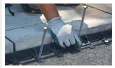
Alliance Gator Nails are high quality nails which are available in lengths of 10" (25 cm) and 12" (30 cm), common or spiral models. Gator Nails are designed for use with all Gator Edge types.
