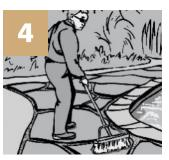
**4** Using a soft, fine-bristle broom, sweep all excess GATOR DUST off wet cast or natural stone surfaces. Ensure that GATOR DUST lies at least 1/8" (3 mm) below the top of the wet cast or natural stones or erosion may occur.
