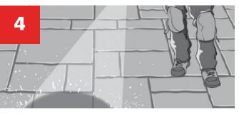
Shower for a minimum of 30 seconds for 30 sq. ft. (3 sq. m.) or until the GATOR MAXX **G2** repels the water and the water starts to accumulate on the joints.
