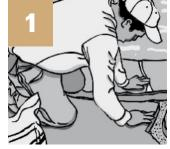
**1** Install the wet cast or natural stones on a maximum 1" (25 mm) bed of sand. Make sure that there is at least 6" (15 cm) of compacted crushed stone under the bedding sand. See diagrams below.
